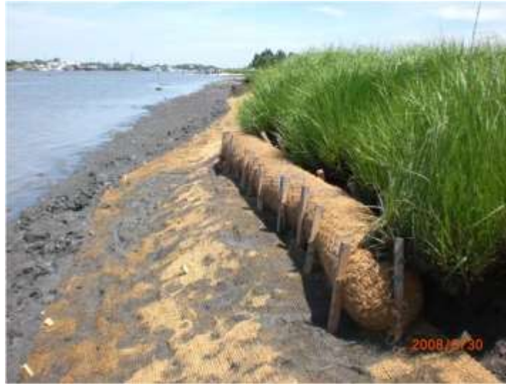
Figure 2-8. Coir Logs and Mats
