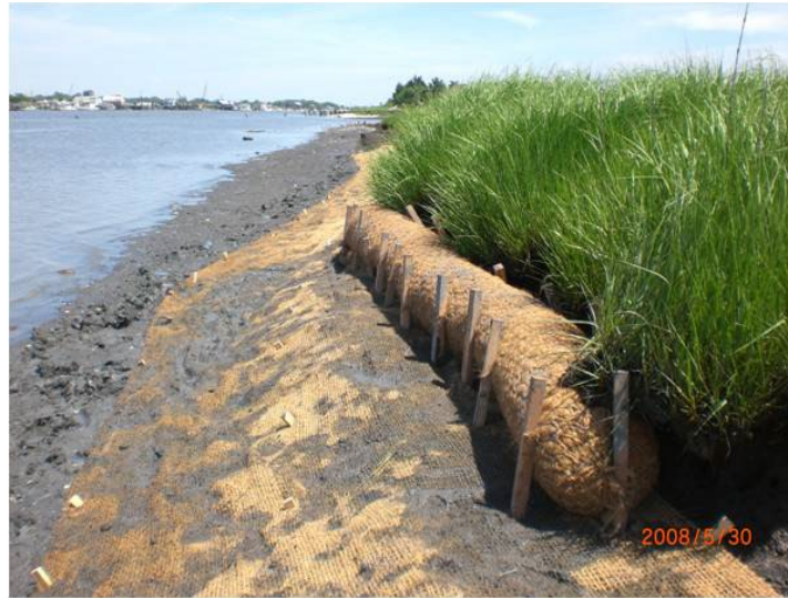
Figure 2-8. Coir Logs and Mats
